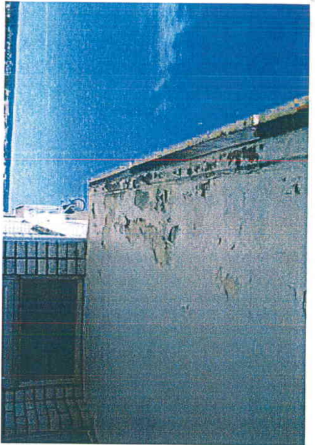
B25. peeling paint on balcony slab soffit.
