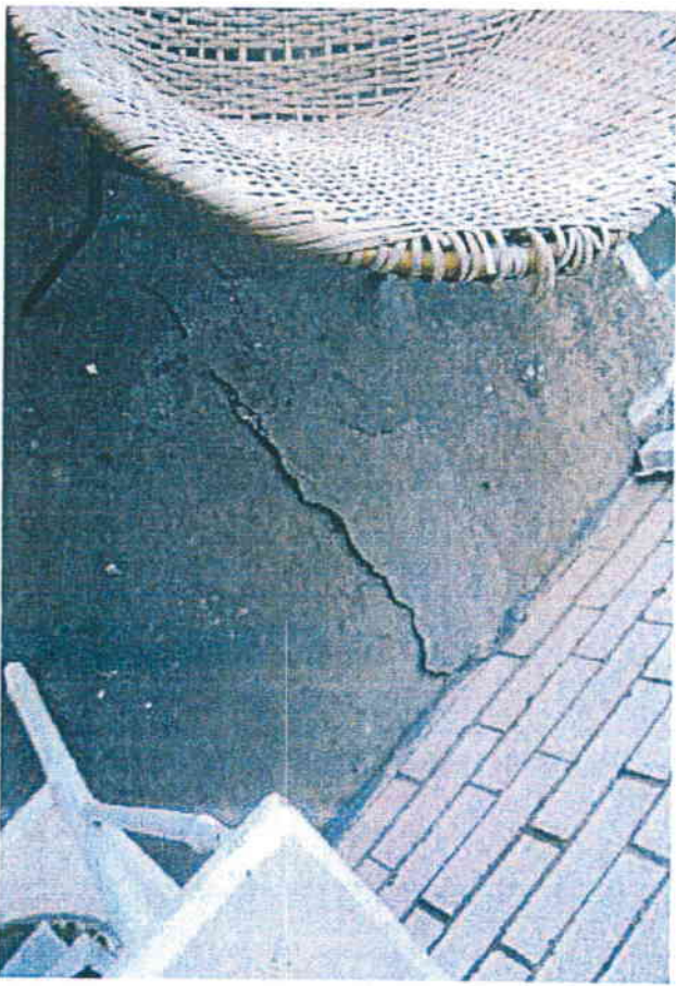
B24. Delaminated concrete on balcony slab at previous repair.
