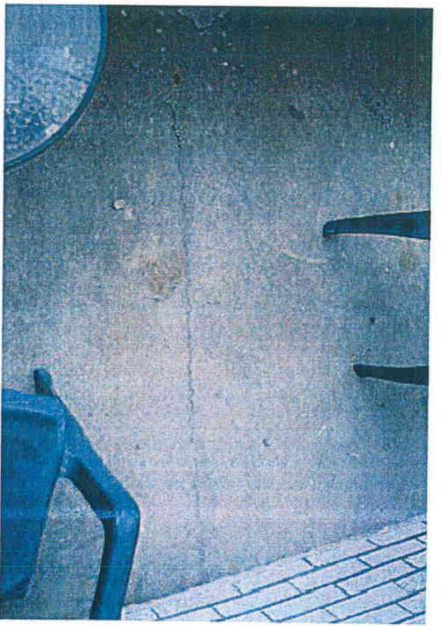
B26. Crack in balcony slab.
