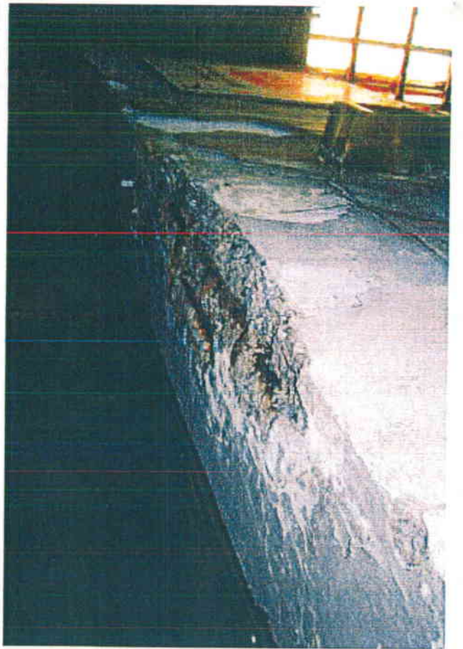
B21. Spalling at garage entrance.
