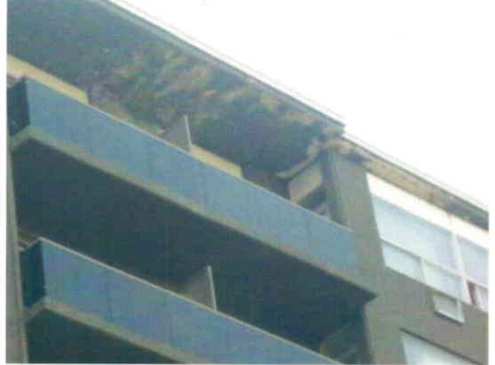
Paint loss (north side)
