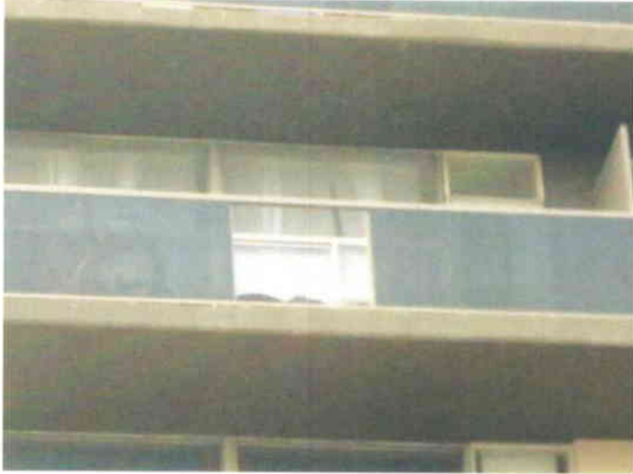
Broken glass panel (front)
