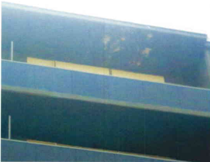
Paint loss (north side)
